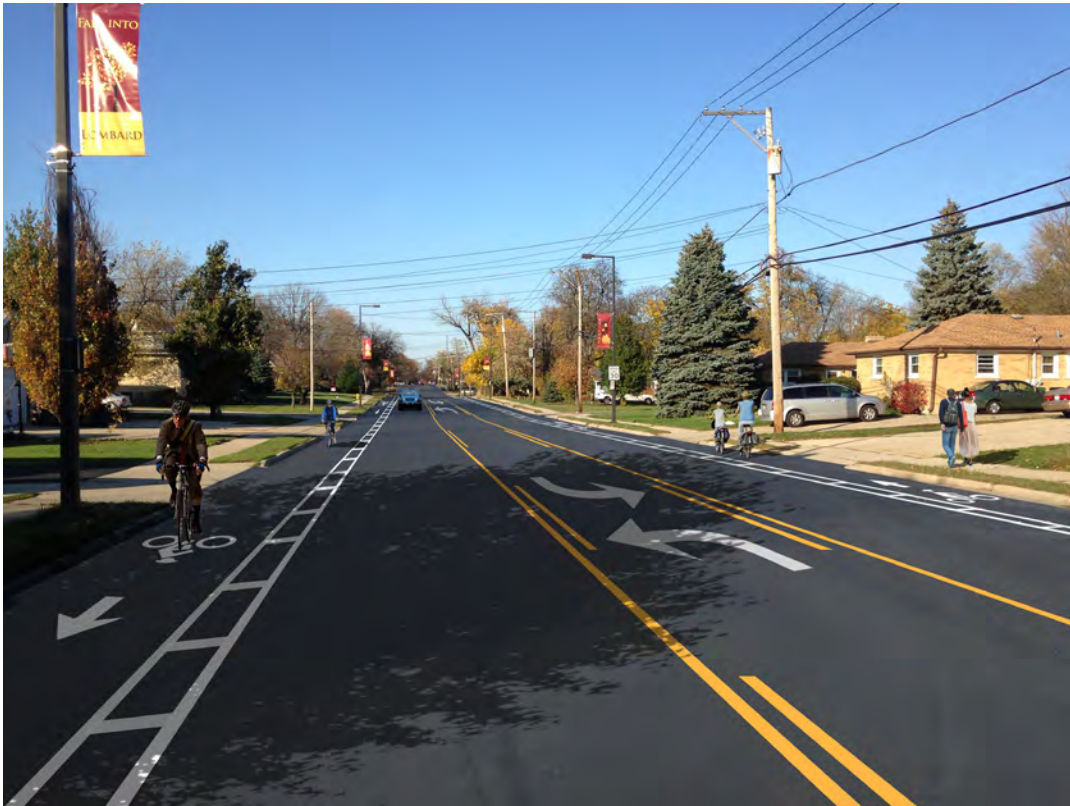
Figure 56. A photosimulation depicting Westmore-Meyers Road following a reallocation of travel lanes. The proposed design includes bike lanes and a center turn lane.
