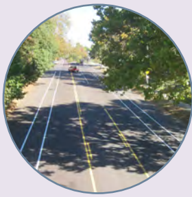
Right-of-Way Reallocation ("Road Diet")
