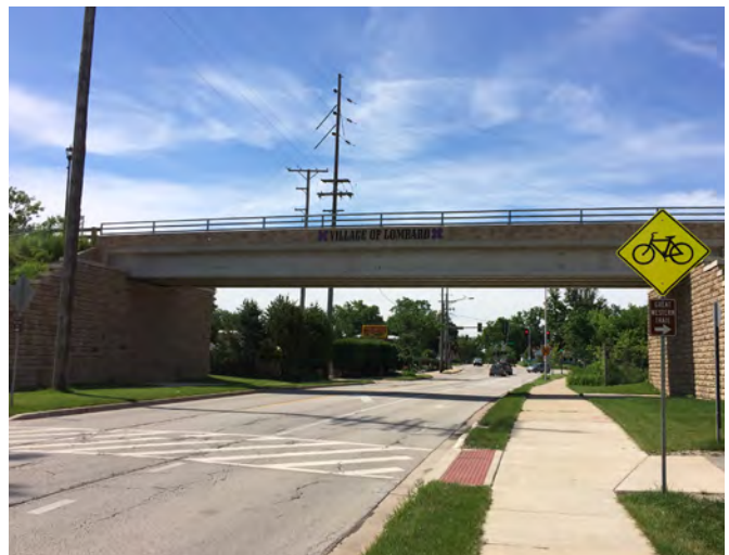
Great Western Trail Pedestrian Bridge crossing over Grace Street
