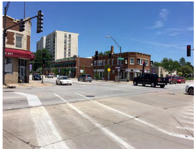
Intersection of Main Street and St. Charles Road with angled crosswalks and wide curb radii
